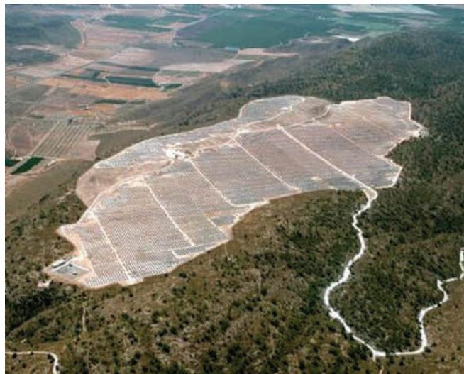
**Bolthouse Farms-** 1.9 Megawatt Solar Power System in Palmdale, California. Designed and installed by Regenes Power, LLC using 10,300 high-efficiency solar panels from Mitsubishi Electric, the new ground-mounted photovoltaic solar arrays employ a tilted single-axis tracking system that follows the sun during the day for greater efficiency—maximizing energy production.
